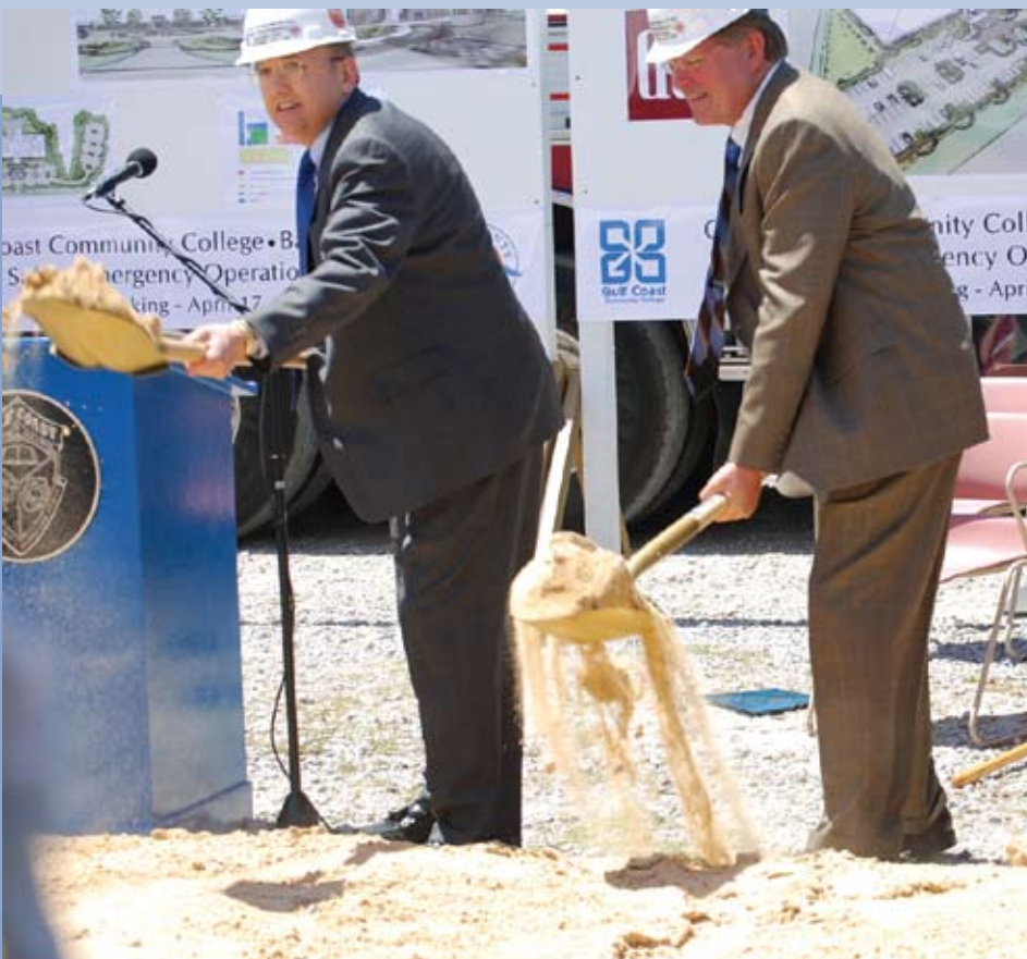
Bill Cramer, chair, District Board of Trustees (left), and Dr. Jim Kerley, president, officially break ground for the Emergency Operations Center at the North Bay Center.
